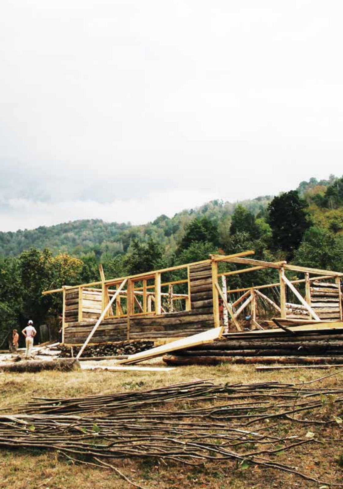
*During construction work on the main building, the craft knowledge of our Romanian hosts came to the fore, and we all observed and tested methods of cutting and joining timber using hand-tools and chainsaws, including low-tech methods to achieve precision of workmanship, such as using a plank nailed to a log to serve as a guide for cuts made using the chainsaw.*
